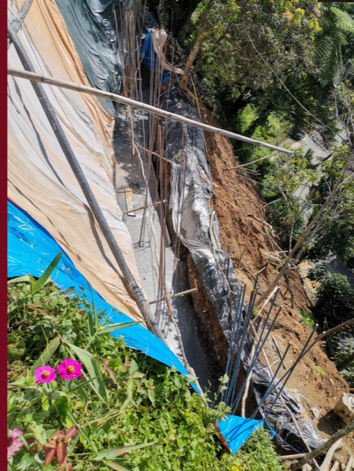
Stonewalling project was started to preempt possible collapse of driveway and ramp at southern part of the hospital. The ramp is the only access-way to the 2nd floor for stretcher-borne patients.
